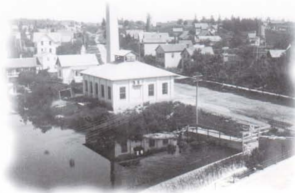
Original steam generators in light plant on Mequon Avenue in the early 1900's.
